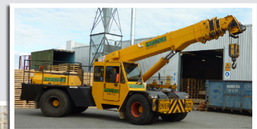
The 20 tonne crane used to lift the steel container and hose.
